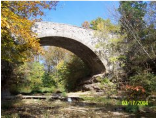
Your Bridge to the Future
